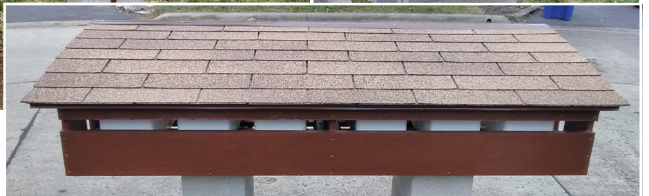
Contemporary lightweight design allows better airflow for less wood deterioration. Concrete pillars create a low-maintenance support structure.
